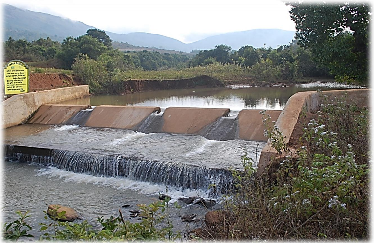
Check Dam at Thuria, G.P: Kotia, Block: Pottangi by Watershed
