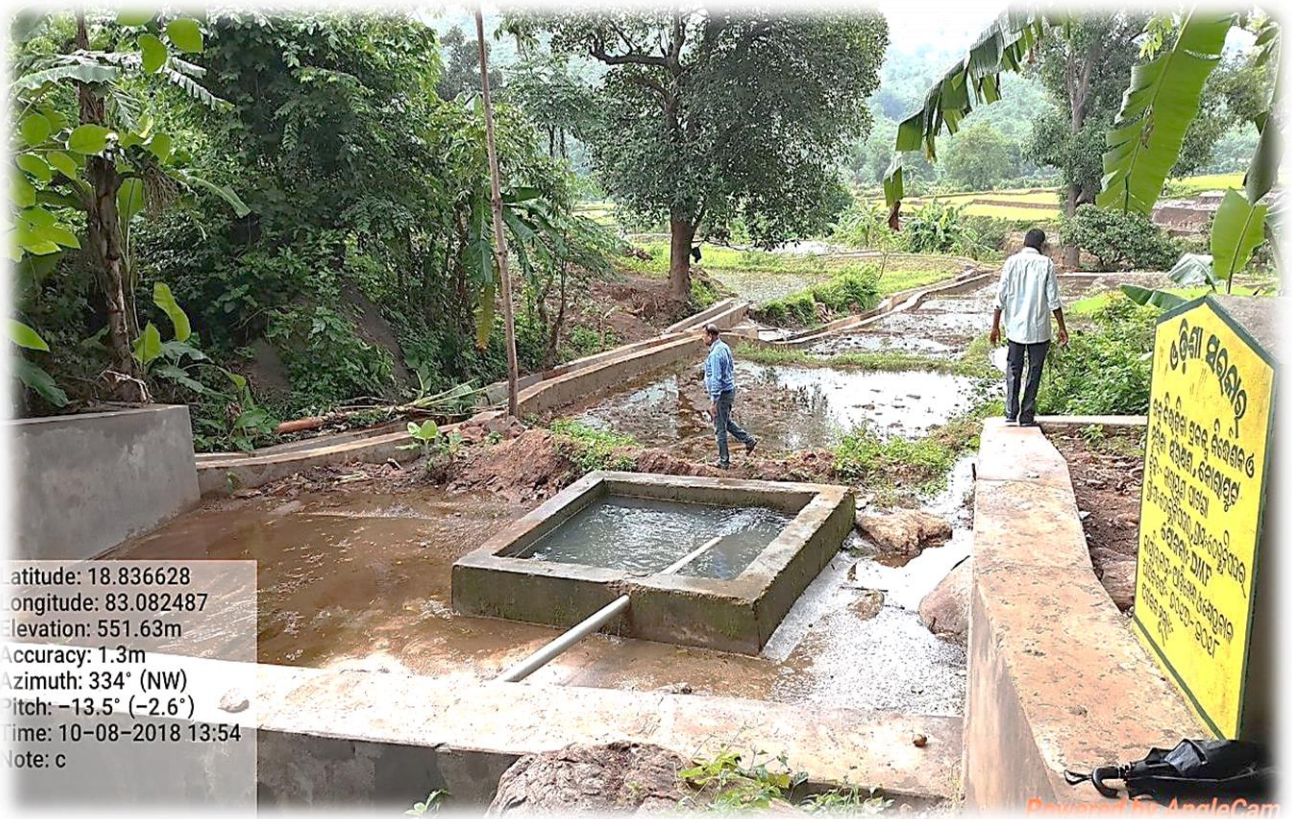
Diversion weir & field channel at Tentulipadar of Narayanpatna by Watershed
