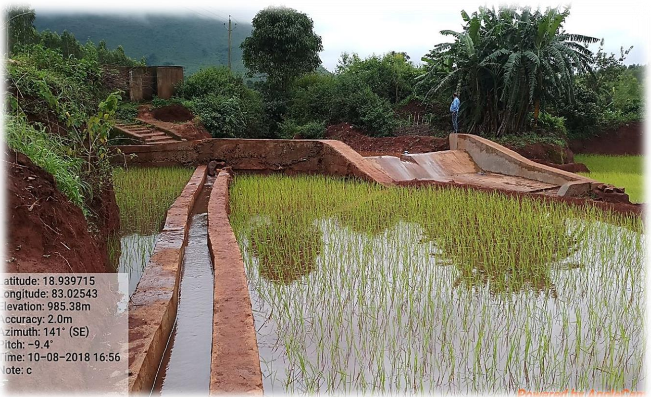
Diversion weir with filed channel at Kudipadar of Laxmipur block by Watershed
