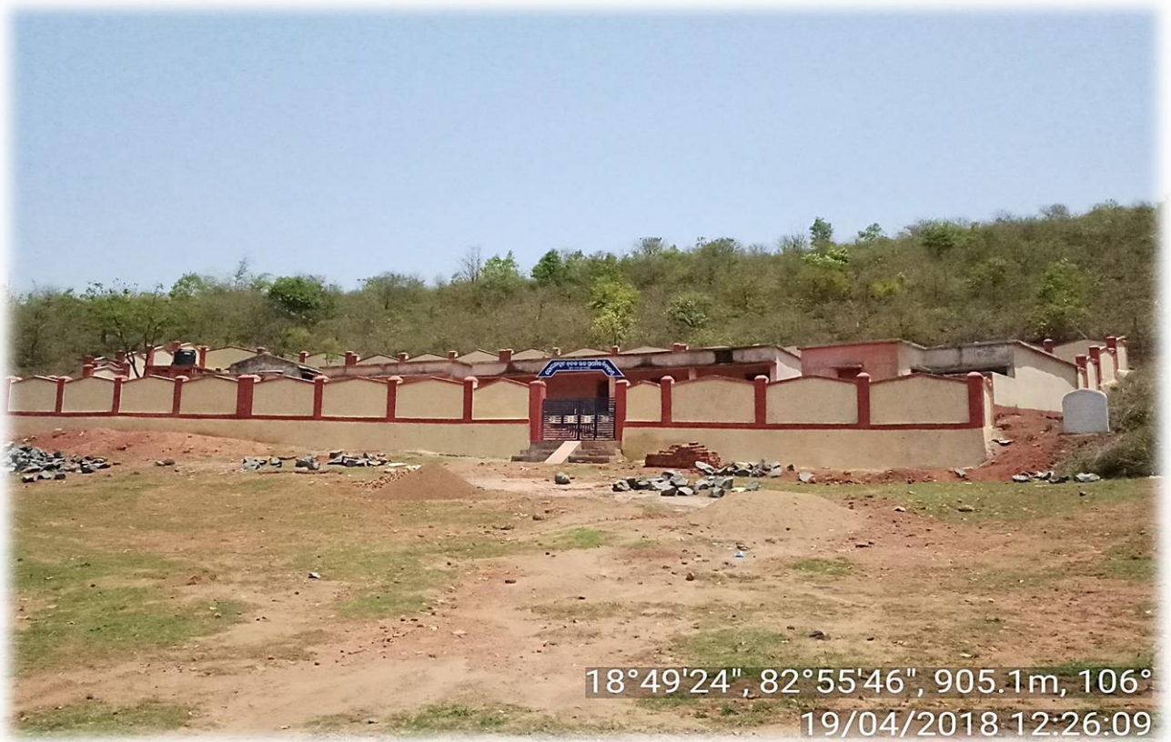
Kankadaput (Boundary Wall), Dasmantpur Block by SSA
