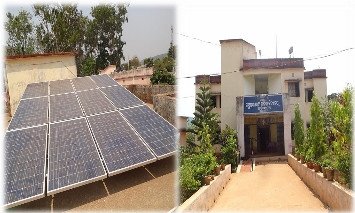
Solar Lighting at SSD/KGVV School
